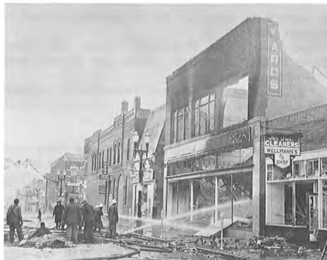
Montgomery Ward Store and Mix Cleaners fire - 1947
