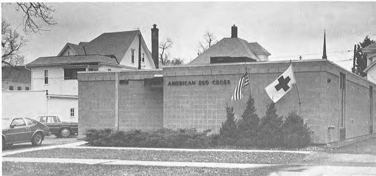
Mower County Chapter, American Red Cross Headquarters Building, 305 NW 4 Avenue, Austin, Minnesota, completed in October of 1973 and dedicated on May 17, 1974.
