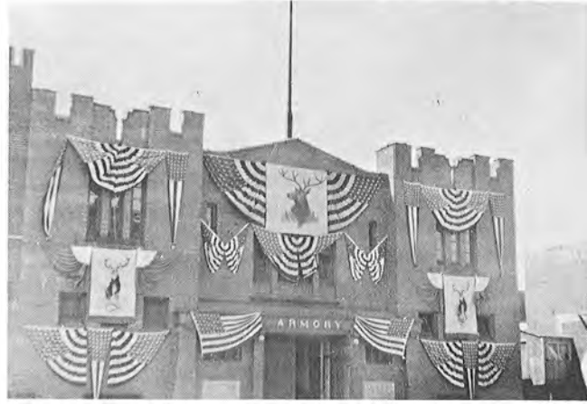
Armory Served Over Fifty Years Dedicated in September, 1912, this armory on 1st Ave. N.E., Austin, gave good service until October, 1963.
