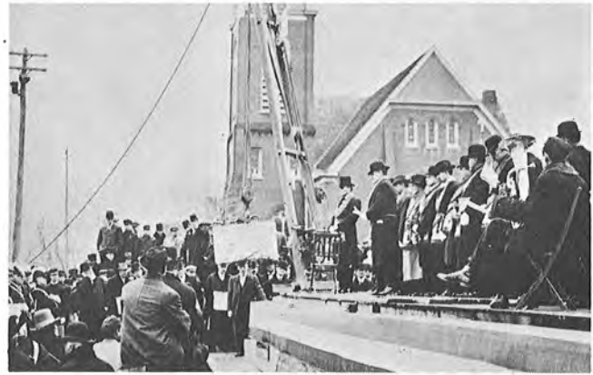
Laying of the cornerstone for a new post office in 1910. The building was completed in 1912. St. Olaf Lutheran Church in background.
