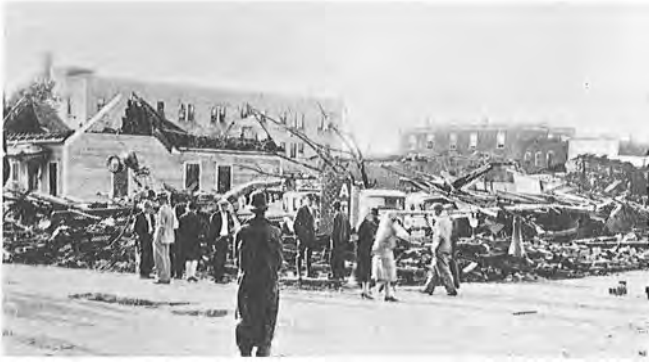
The tornado destroyed the Motor Inn at the corner of Water St. and Chatham St. (4th Ave. N.E. and 1st St. N.E.) A newly hired mechanic, August Neubauer, died when the building collapsed.
