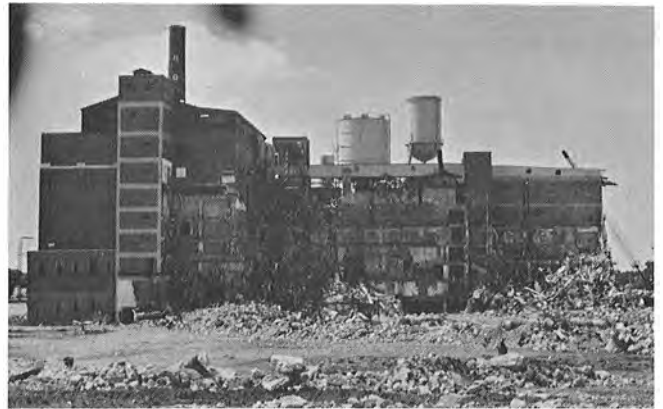
Old Hormel Plant, closed in 1982, continued to be demolished in 1984.
