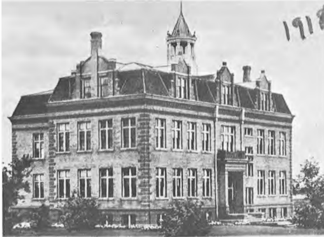
University of Southern Minnesota - main building
