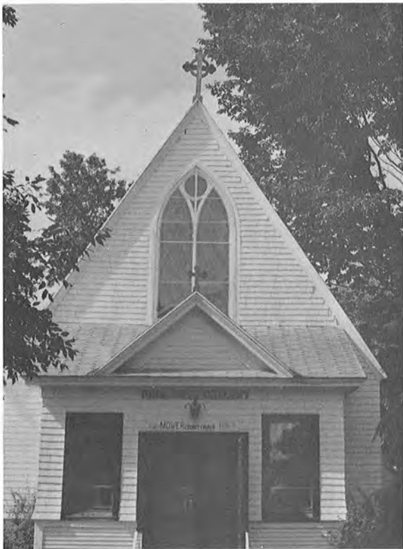
Early church Now Fine Arts Gallery This was formerly the Christ Episcopal Church, Austin, given to the Historical Society by Mr. and Mrs. H. E. Rasmussen.
