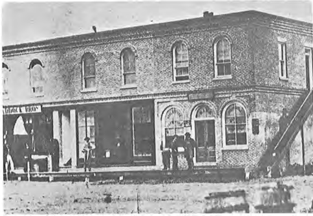
First National Bank Building rebuilt after 1869 fire
