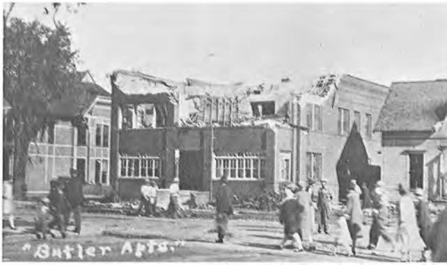
Butler Apartments following 1928 tornado
